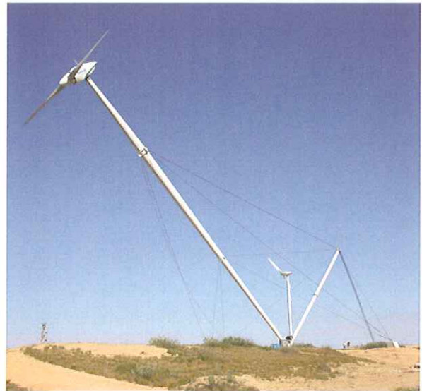
Wind turbine being lowered.
